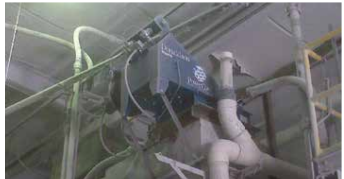
CPV-2 - Day bin with porcelain dust 800 cfm (1,359 m 3 /h)
