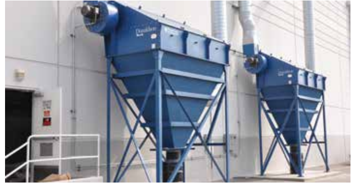
CPC-24 - Paper tissue manufacturing 7,600 cfm (12,910 m 3 /h)
