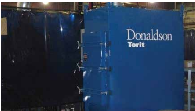
TG4 on Welding
