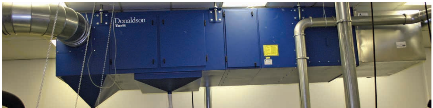
MODULAR MEDIAFILTER™ on Grinding 2,000 cfm ( 3,397 m 3 /h)
