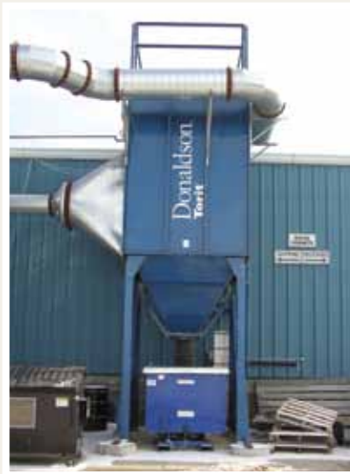
54MBTH8 at a cabinet shop on wood dust, from cutting, moulding and sanding
